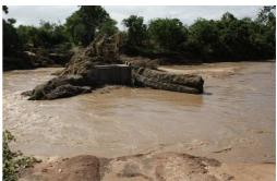
This erosion was expected and an integral part of the design of the bridge. The bridge itself has virtually no damage and the process of rebuilding the approach and departure roads to the bridge is well underway.
